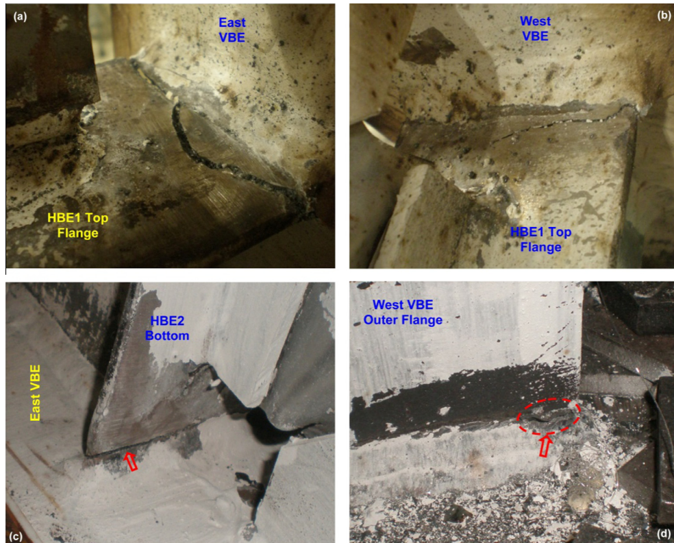
Fig. 5. Special-moment resisting connection fractures in displacement Step 10c ( \Delta_3 = 3.33\% drift = 7.09\delta_y ): (a) and (b) HBE1; (c) HBE2; (d) West VBE.
